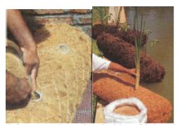
CoirLogs can be equipped with prefabricated planting holes.
