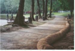
CoirLogs trap the downslope sediment, minimizing siltation at toe of slope.
